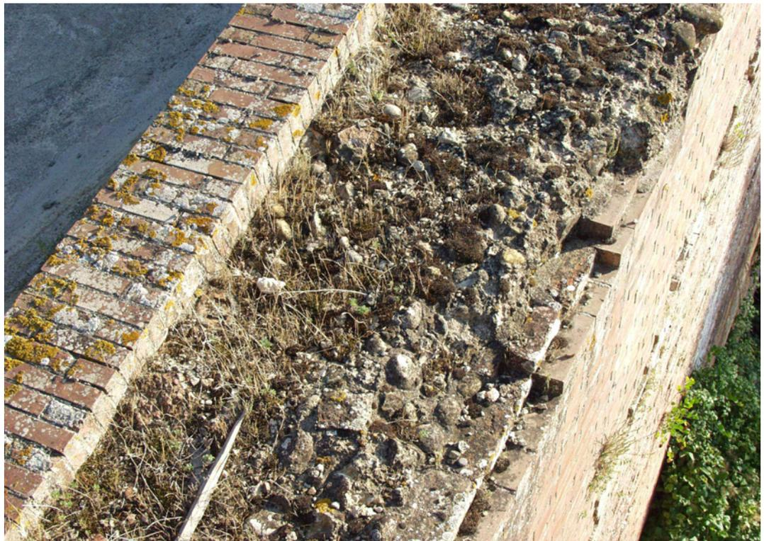
Fig. 6 - Typical construction "a sacco" of the city walls of Siena.
