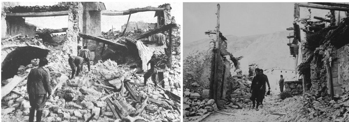
Fig. 1 - View of the collapse of some poor stone-masonry houses in a village east of the Maiella Massif (left; L'illustrazione Italiana, 1933) and in Lama dei Peligni (right; photo Keystone-France/Abruzzes/gettyimages).
