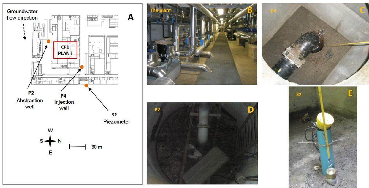
Fig. 5 - Open Loop System (GWHP) installed in the “Politecnico di Torino” for cooling some of the university buildings. Schematic map with location wells and piezometer (A), the heat pump plant (B), P4 is the injection well (C), P2 is the extraction well (D) and S2 is the piezometer located towards respect the wells (E).
